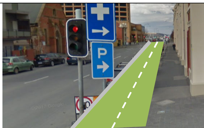
Example of separated cycleway treatment on block between Collins and Macquarie St.
